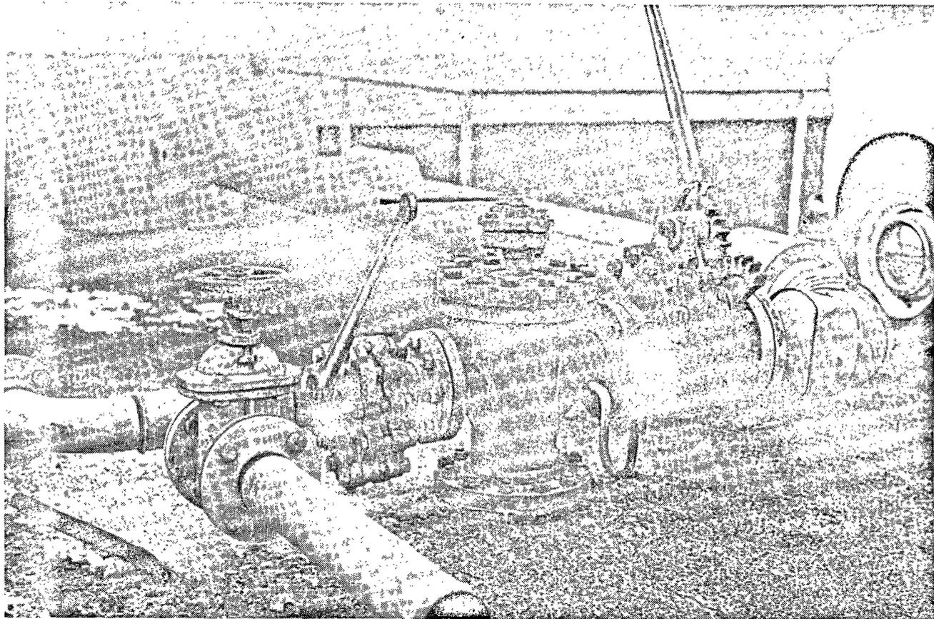
Figure 7. 6" well-head with 4" branches at Rotorua Hospital
