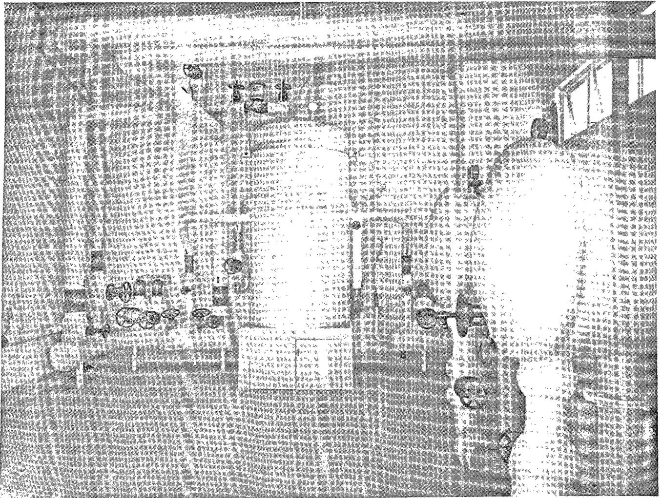
Figure 8. Heating and hot water supply exchangers at a hospital
