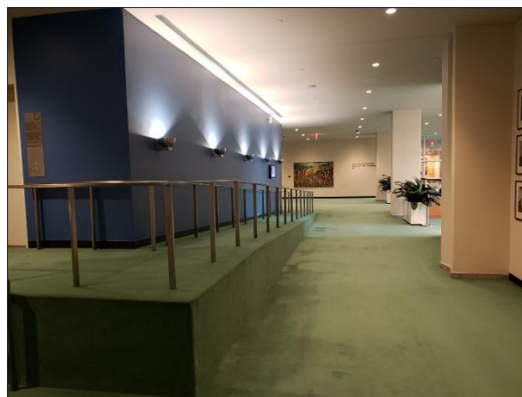
GA-200 accessibility ramp. Source: Department of Operational Support/Facility and Commercial Activities Service
